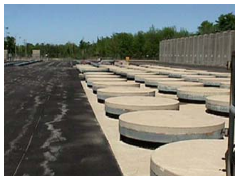
Figure 1.b. ILRW in ground storage structures Source: Ontario Power Generation
