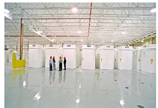
Figure 1.c. Dry storage containers for used nuclear fuel (HLW) Source: Ontario Power Generation
