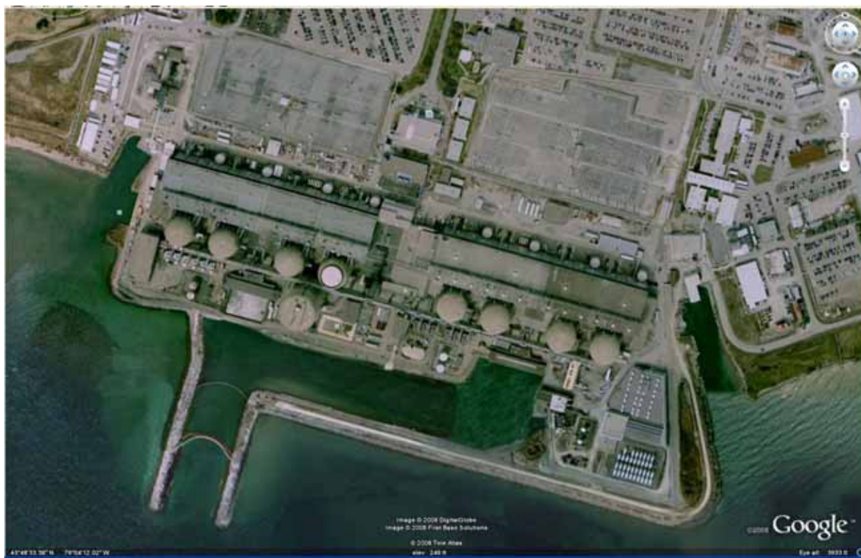
Satellite Image of Pickering Nuclear Generating Station (Image: Courtesy of Google Earth)
