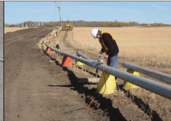
Image #6: NDT pipeline inspection, using industrial radiography equipment
